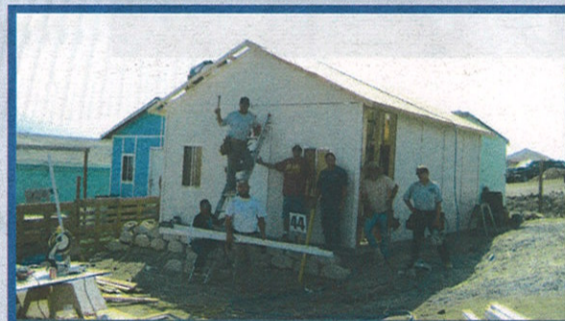
Whitaker Investments and Hamann Construction
